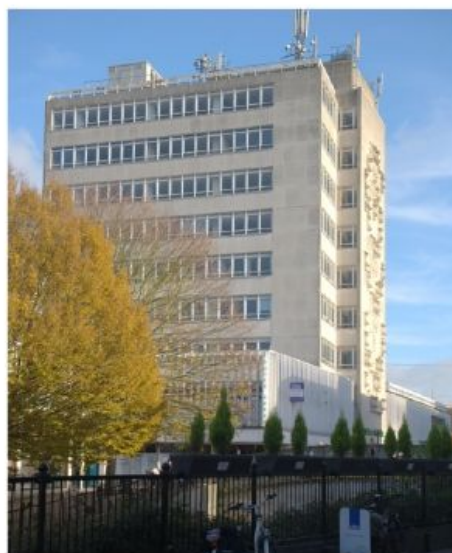
CANSIDE Cater House Chelmsford (Completed)
