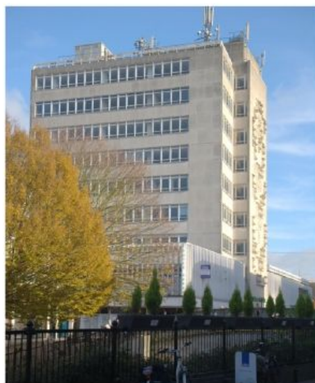
Cater House Chelmsford (Completed)
